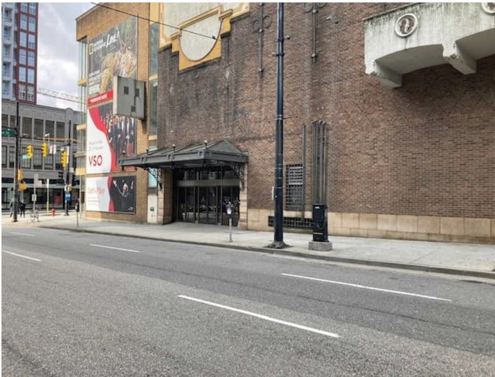
Street Bus Parking With Shore Power Box
