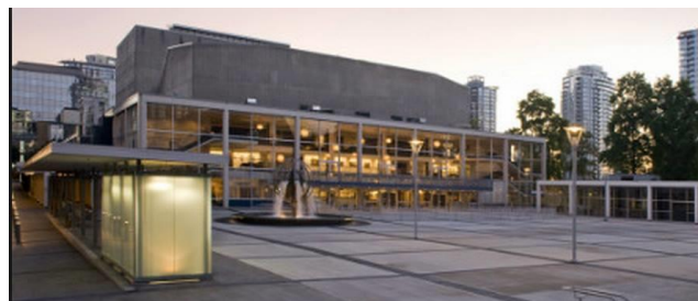
Figure 4 šxʷálexən Xwtl'a7shn (formerly QET Plaza)
